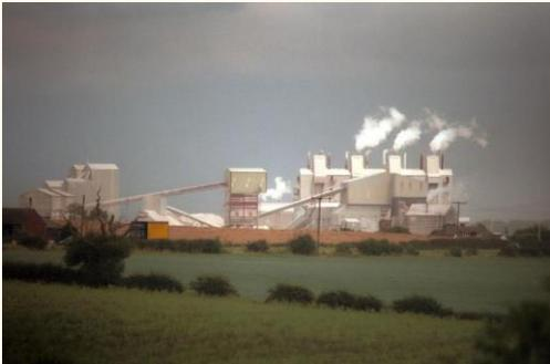
Firstly, raw materials are quarried and transported to a cement facility. These materials would include lime, shells or chalk, silica or fly ash from coal combustion, alumina from clay or shale or fly ash from coal combustion and iron oxide from iron ore or from iron containing by-products.
